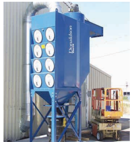
DFO on Plasma Cutting 5,000 cfm (8,493 m 3 /h)
