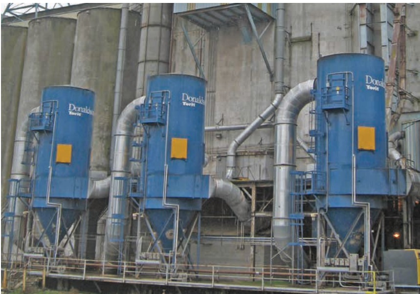
RF - Grain Terminal 61,000 cfm (103,618 m 3 /h)
