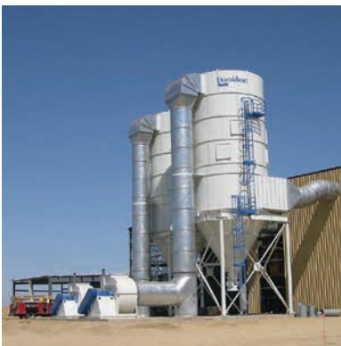
LP on Nut Dust 280,000 cfm (475,622 m 3 /h)
