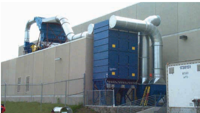
DLMC on Paper Dust 27,000 cfm (45,864 m 3 /h)
