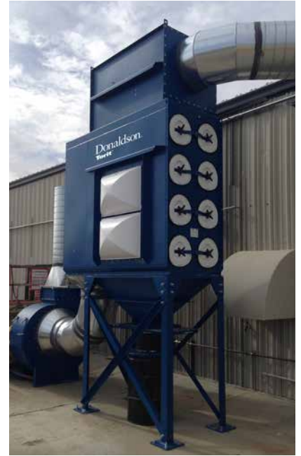
DFO on Plastics Routing 16,000 cfm (27,184 m 3 /h)
