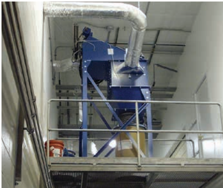
CPC on Milk Powder 1,200 cfm (2,038 m 3 /h)
